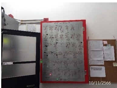
Graphic Annunciator Fire Alarm System
